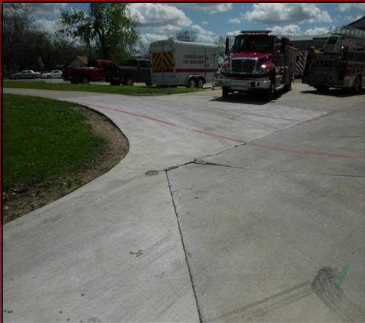
The parking area and apron area at Central Fire Station received \$11,280 in improvements funded by tax notes. Due to wear and tear, all identified concrete and pavement was replaced with thicker concrete in accordance with the current building code.
